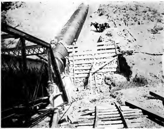
FIG. 5.—WOODEN STAVE PIPE ON WEST BRANCH AND END OF BRIDGE.
